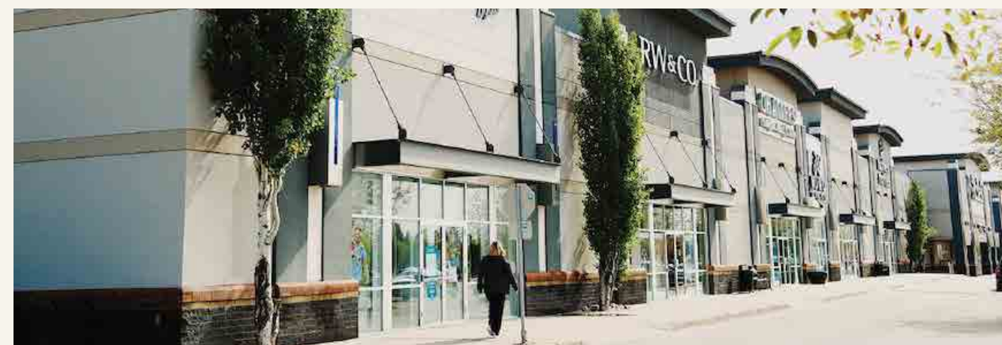
Skyview Centre, AB
